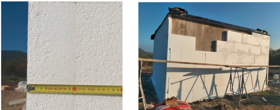
Abb2: Installation der EPS Dämmung Austrotherm AT-H80 Figure 2: Application of the EPS insulation Austrotherm AT-H80
